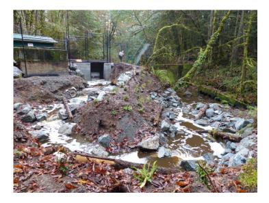
The Tod Creek fishway is about 30 metres long and functions like a ladder with "step pools" to help the fish around a dam. Photograph By Submitted
