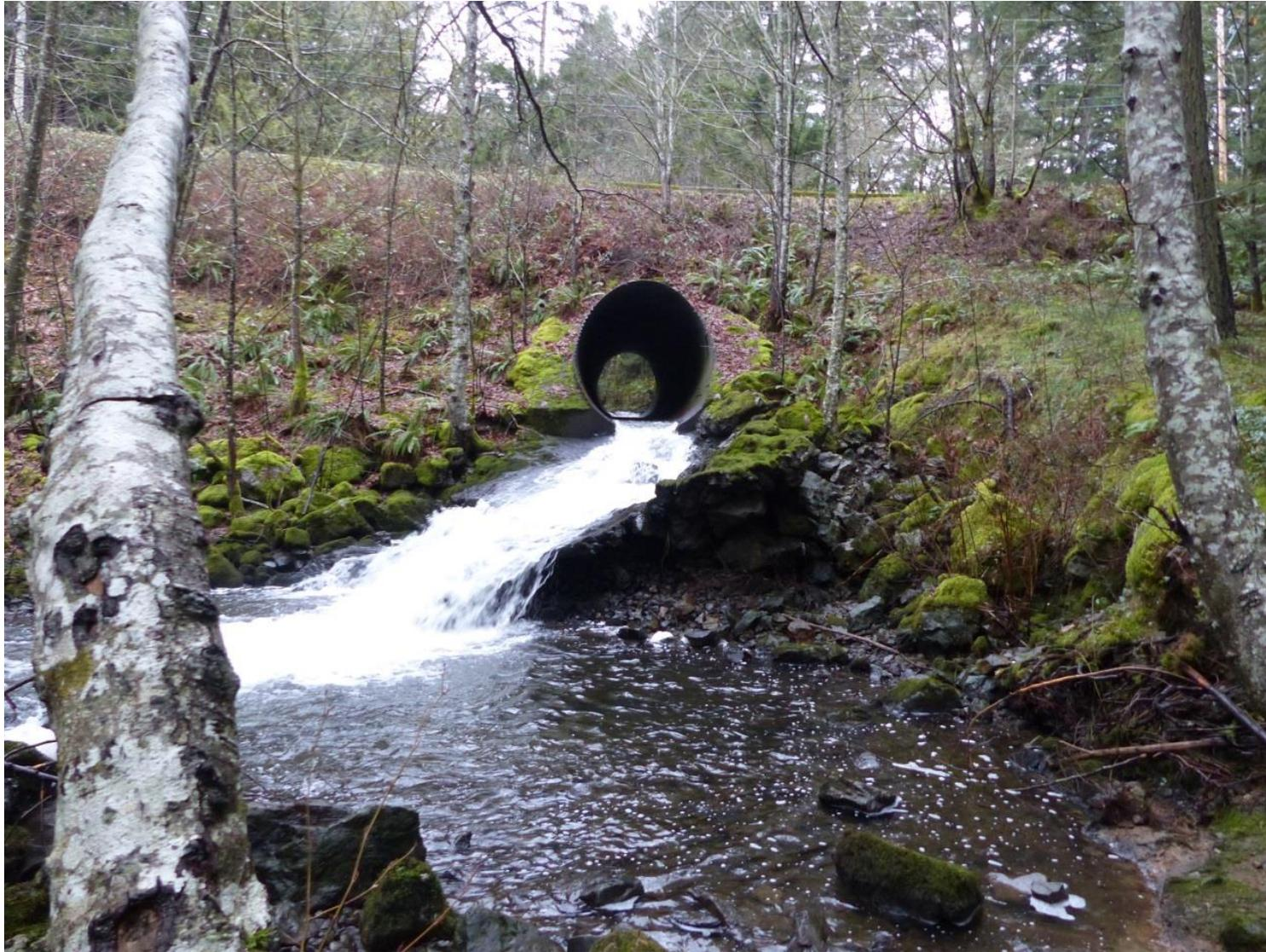
*Figure 3. Millstream Creek at the Atkins Road culvert, the barrier to fish migration.*
