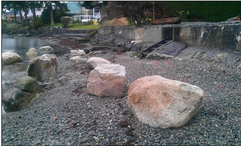
Figure 27. Image of seawalls in the supratidal zone of Roberts Bay, as well as some large boulders that were placed on the beach near the Ardwell Avenue public access point (image courtesy of Adrian Rowland, year unknown).
